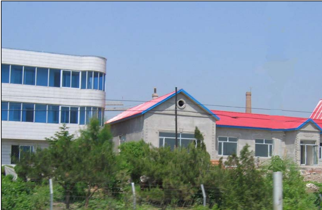
New houses under construction in rural areas of Longjin.
