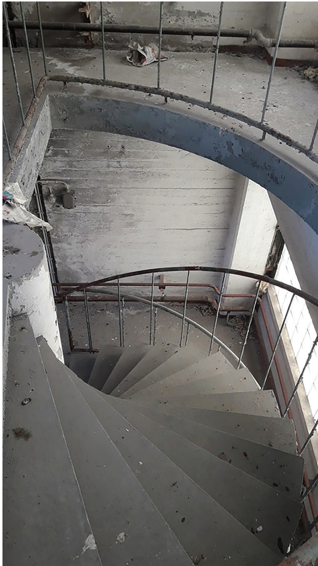
Figure 3. Stairway in an abandoned factory. Photo by Vesa-Pekka Herva.
