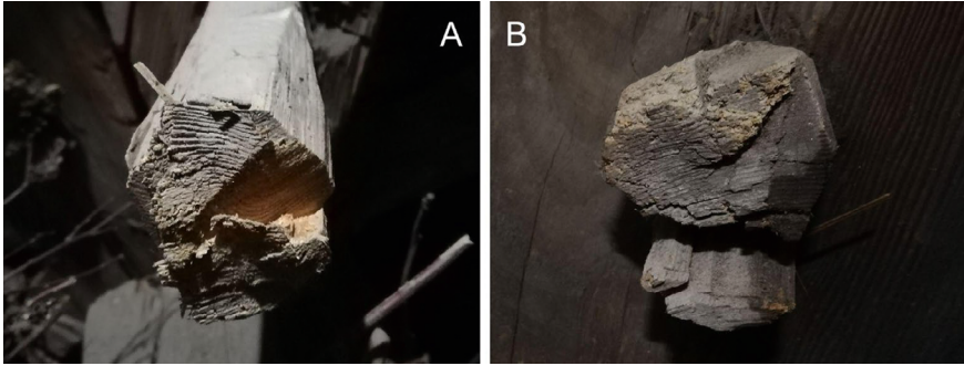
FIGURE 11 Dowel profiles in Pyhtää Church with a different wood grain pattern © FRANZISKA DALHEIMER (2023)
