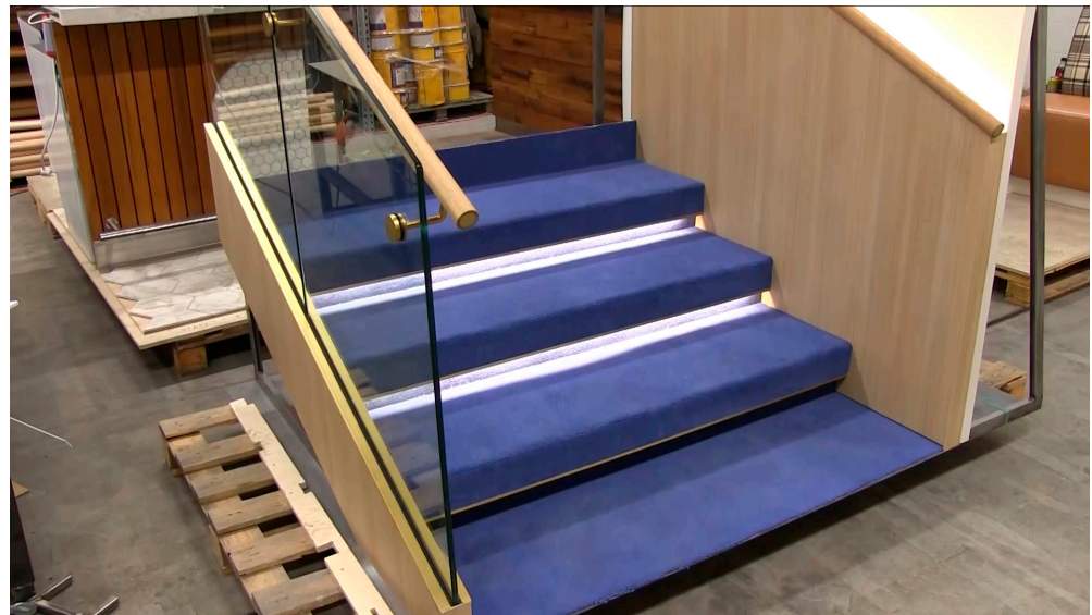
Figure 2. An example of a physical mock-up. This piece of a staircase was built for verification of the appearance and build quality before beginning the construction of the actual interior.
