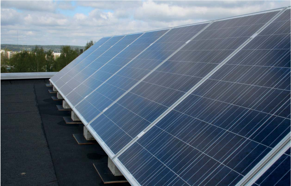
Figure 2: The first panel string installed
