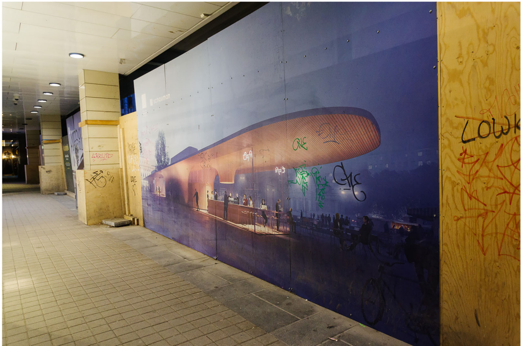
Figure 2. Schauman & Nordgren Architects' vision of TMS (as seen on Kauppiaskatu). Photograph taken by author.
