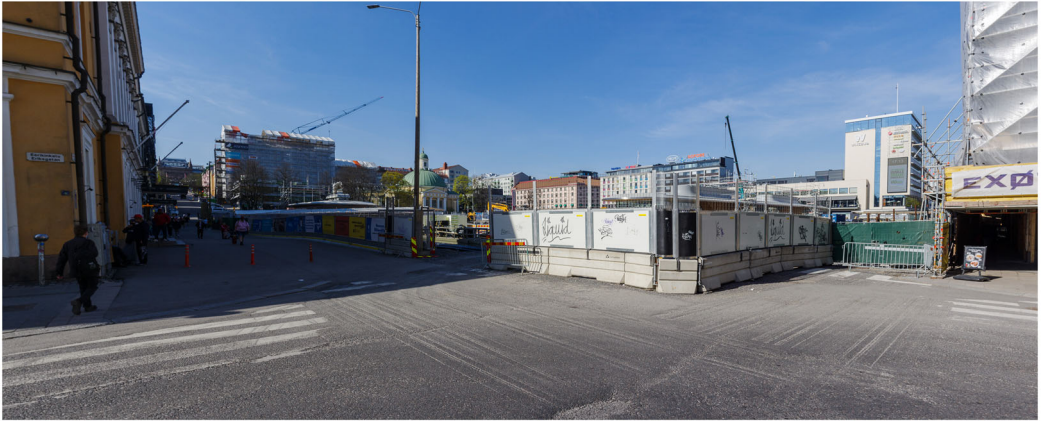
Figure 8. TMS in daylight (view from the corner of Aurakatu and Eerikinkatu). Source: Photograph taken by author.
