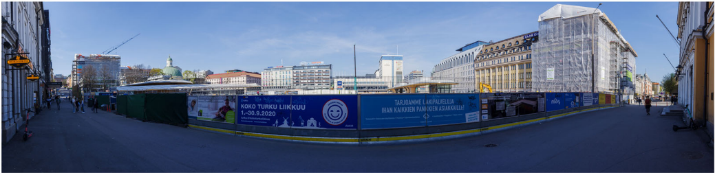
Figure 6. TMS in daylight (view from Aurakatu). Source: Photograph taken by author.
