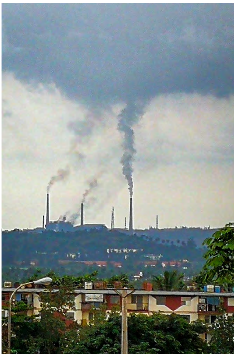
An industrial power plant, Moa
